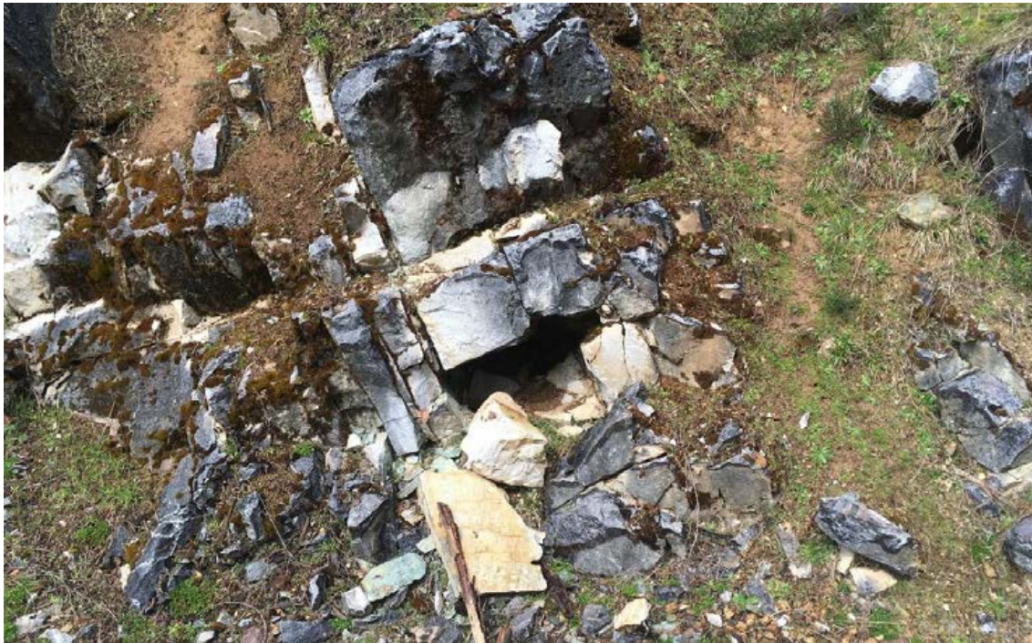
Photo 01: Observed cavity within bedrock slope to the east
